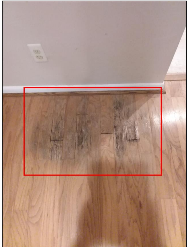
Item 18 - Item 2(Picture) Living room - measured dry
