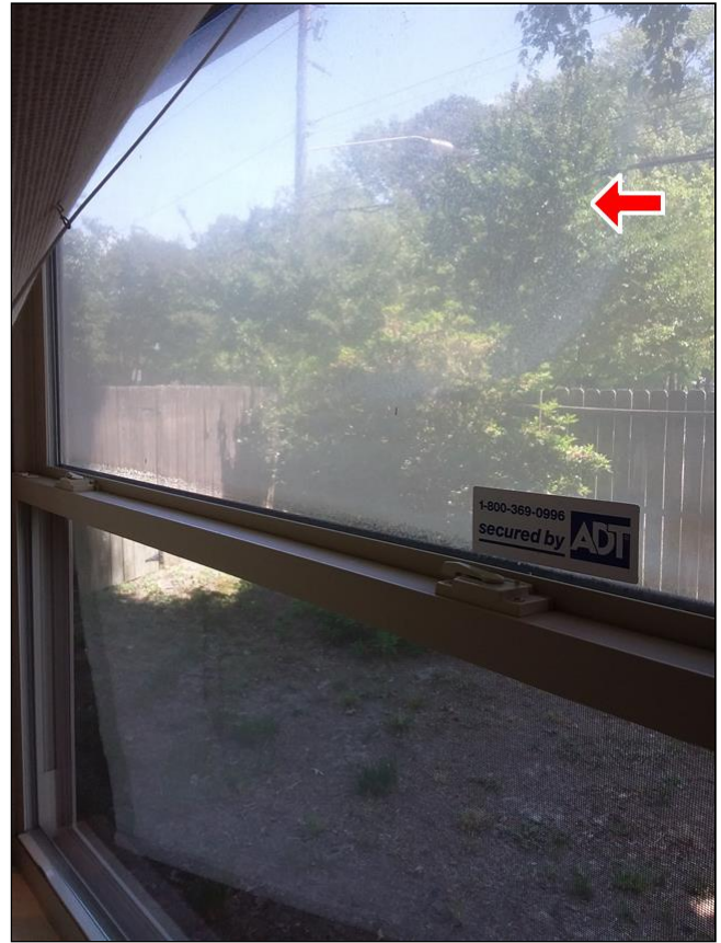
Item 6 - Item 2(Picture) Common room rear wall
